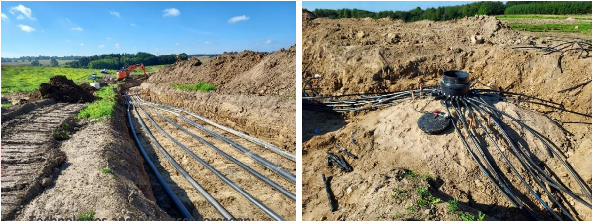
Picture 5. Geothermal heat system extracting ground heat (under construction).
