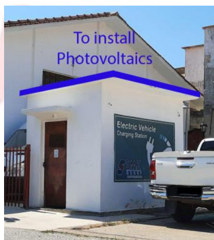
Picture 4. Haldikiki pilot Electrical Commercial Facility for the COMMUNITAS tools deployment.
